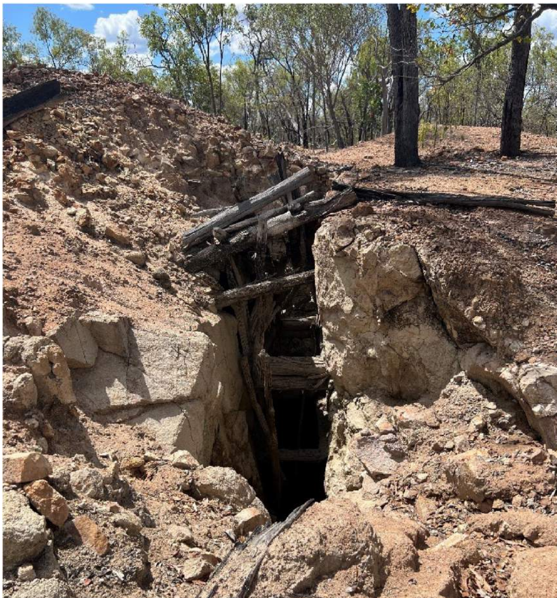
Figure 14 Historical Workings at Frehurst
